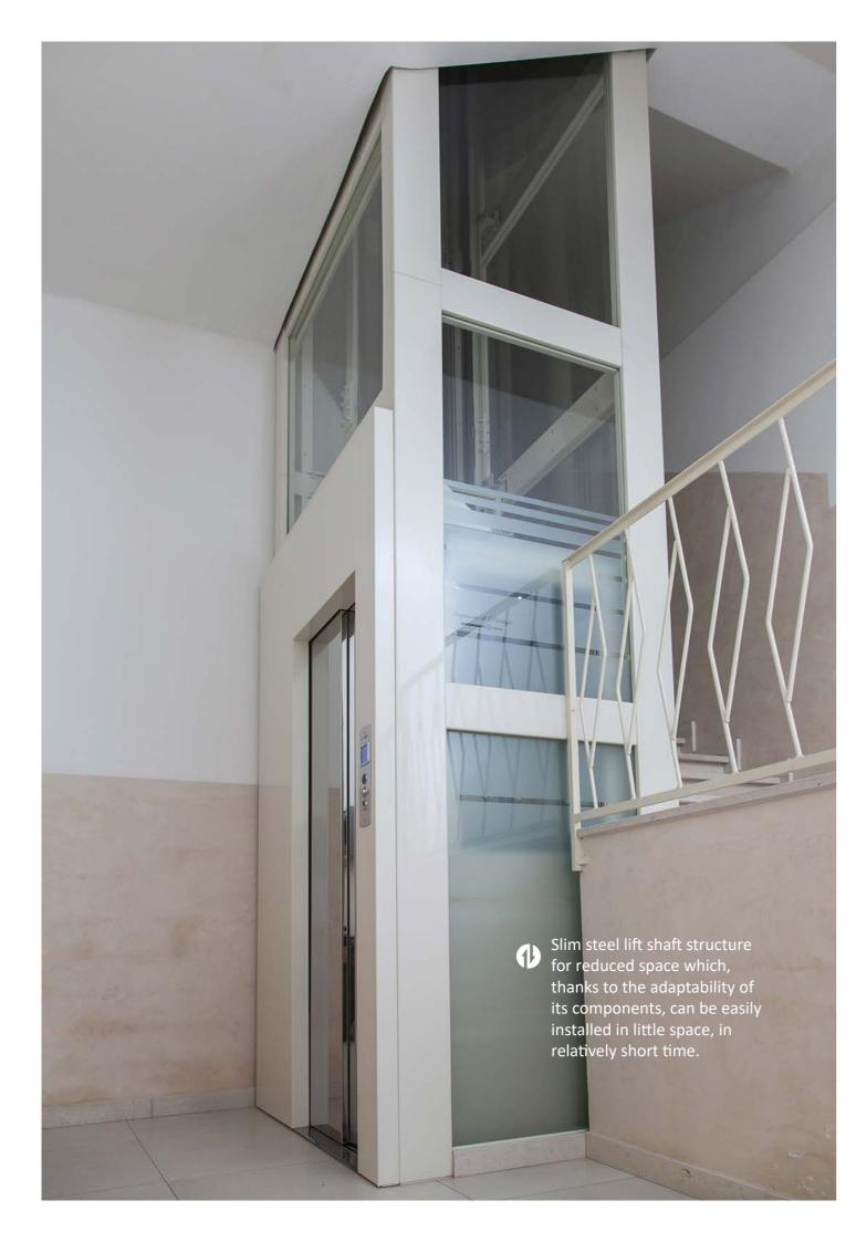
Slim steel lift shaft structures with a manual swing landing door
