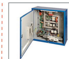
Controller Oil-hydraulic lift plant
